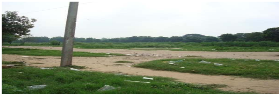
Figure 1- Proposed Site for the Project
